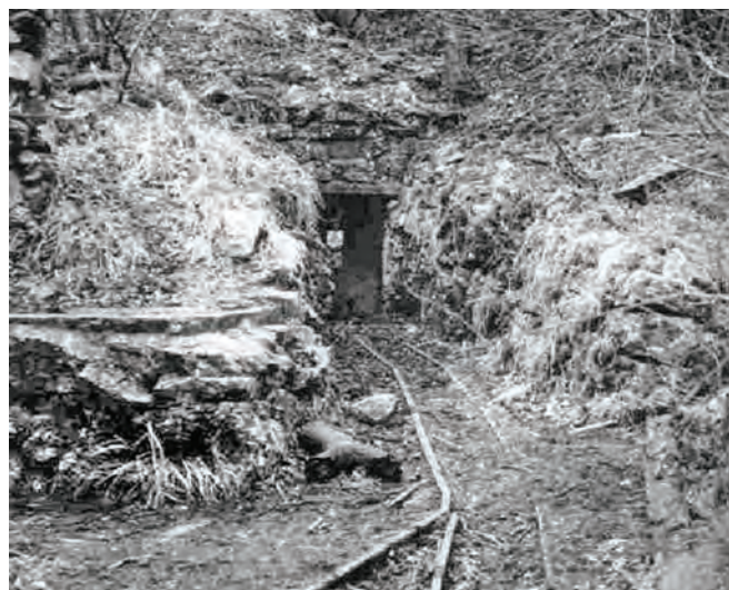
Good Luck mine adit c 1950s
